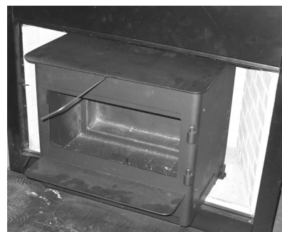
Diagram 5 Pull Rod In Place
